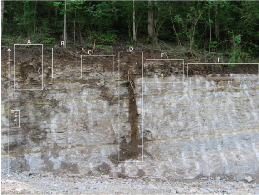
Figure 4. Soil and regolith variability on the Lexington Limestone formation, Madison County, Kentucky. (a) Mollic or umbric surface horizon overlying argillic horizon, and thick transition zone of rock fragments and weathered limestone. (b) Similar to (a), but thinner zone of weathered rock. (c) A horizon directly overlying a thin layer of weathered limestone. (d) Weathered, soil-filled joint with dark surface layer, multiple argillic horizons, and abrupt transition to bedrock. (e) Similar to (c), but greater rock fragment content in surface horizon. (f) Mollic or umbric surface horizon with abrupt transition to bedrock. (a) and (b) are likely Faywood or Salvisa series; (c) and (e) would likely classify as the Cynthiana series; and (f) as Fairmount. (d) would probably be classified as the Maury or Bluegrass series, depending on B horizon clay content.
